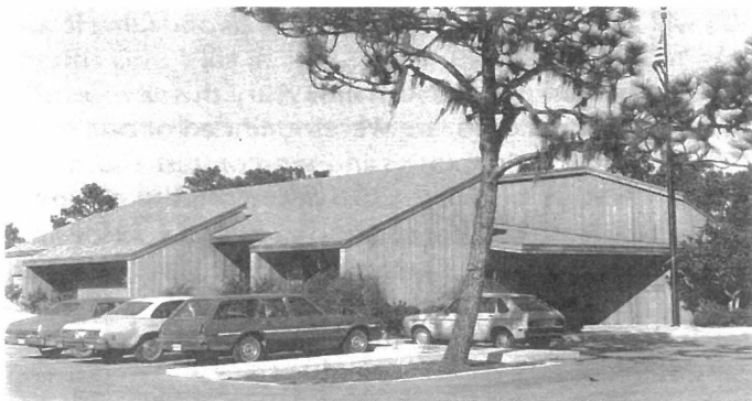
The Youth Ranch administration building was completed in 1979 and dedicated “to the glory of God, in memory of Elmer Ellsworth ‘Dick’ Pilcher, and in honor of his sister, Nancy Pilcher.”
