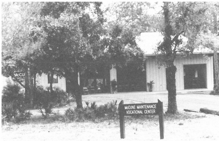
The McCune Maintenance/Vocational Center at Youth Ranch-Bradenton/Sarasota marks the second such building donated by the McCunes. In 1991, a similar building was dedicated at Caruth Camp.
