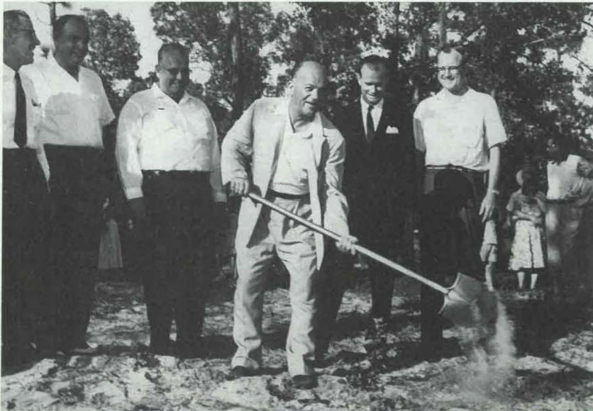
Groundbreaking for the first building at the Florida Sheriffs Boys Ranch was held on August 1, 1958. Acting Boys Ranch Executive Director and Hillsborough County Sheriff R. Ed Blackburn, Jr., took his turn lifting a spade of dirt with a gold-painted shovel and marked the beginning of construction for the first cottage. Joining the celebration and waiting to dig in were (from left) Suwannee County Sheriff Hugh Lewis, Boys Ranch Trustee W. F. Edwards from Dade City, Pasco County Sheriff Leslie Bessenger, Chairman of the Board of Trustees and Monroe County Sheriff John M. Spottswood, and Boys Ranch Trustee J. L. McMullen of Live Oak.
