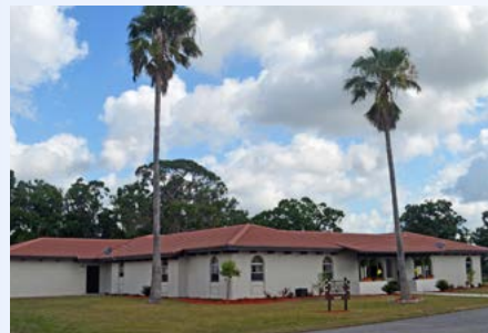
The Polk Sheriff's Charities Scholarship House received renovation inside and out to prepare for the first residents in the fall of 2018.
