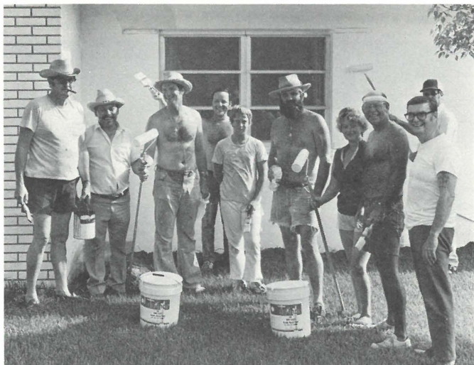
Telephone Pioneers took a two-minute break for a picture before completing a free paint job on the Youth Ranch residence building. Resident Director Joe Spenard took a break with them, then went back to his assignment --- painting shutters with Don Genung, Youth Fund Vice President for Planned Giving.
