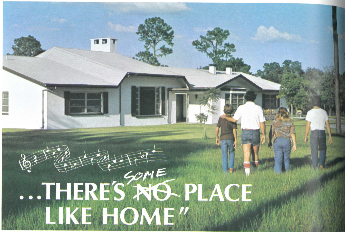
Former Salls home has been renovated for use as the first residence cottage.
