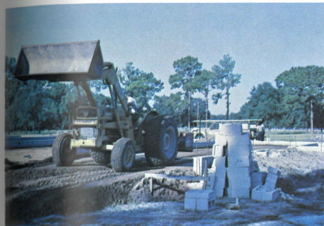
Elmer and Nancy Pilcher Administration Building is under construction.
